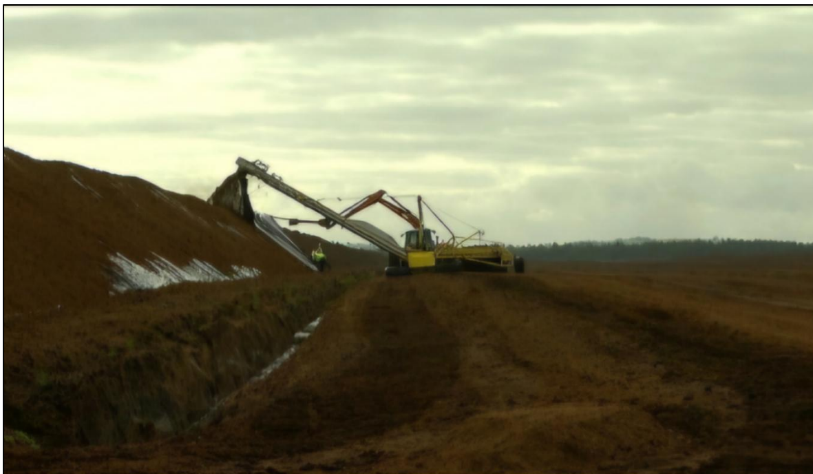
Plate 4-14: Polythene covering of stockpiles
