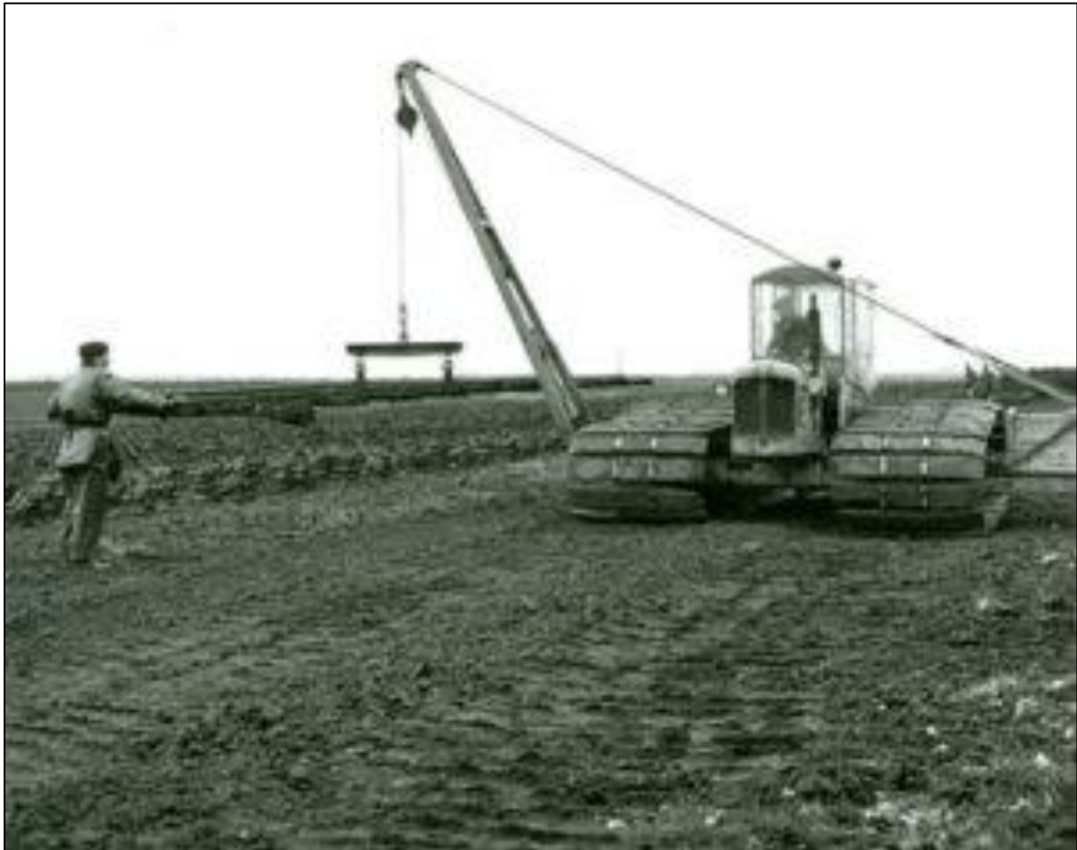
Plate 4-29: Rail moving attachment to lift and lay temporary railway track, along sod peat ricks and milled peat piles. (source: www.bordnamonalivinghistory.ie/equipment-detail/rail-moving-attachment/ )
